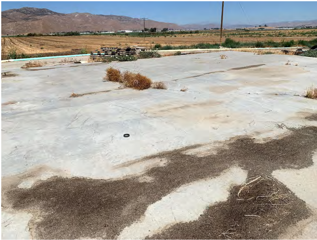
G-21. 100-foot by 50-foot concrete foundation in former residence area (08/03/2021).
