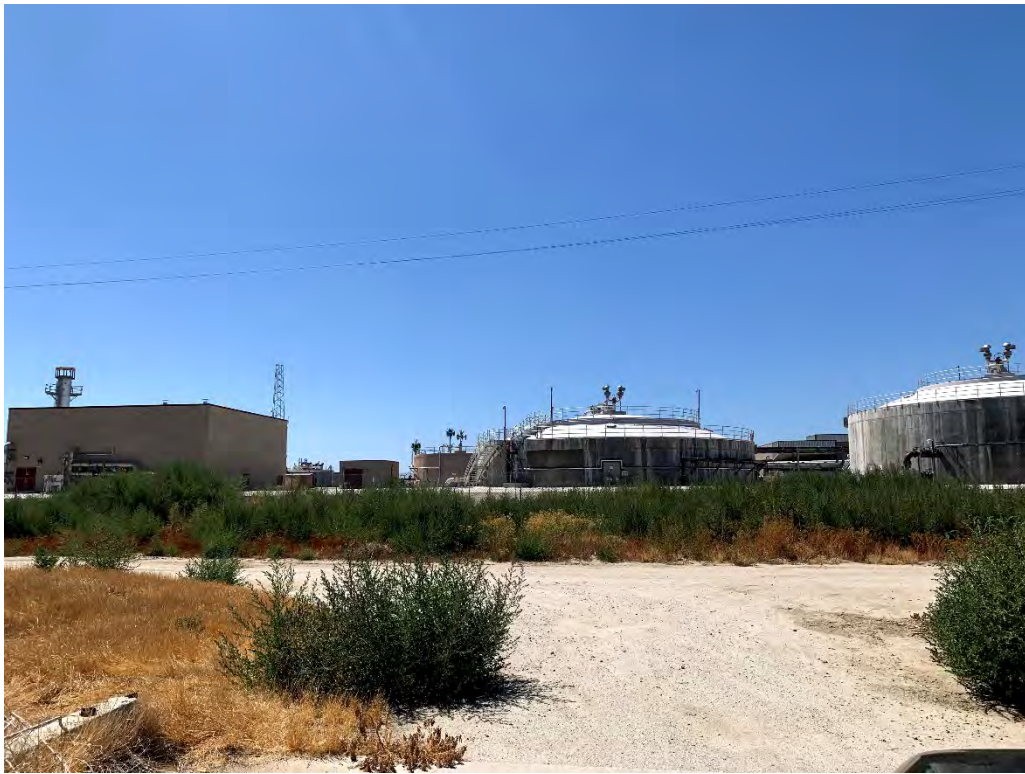
G-29. Southern adjacent water reclamation facility (08/03/2021).
