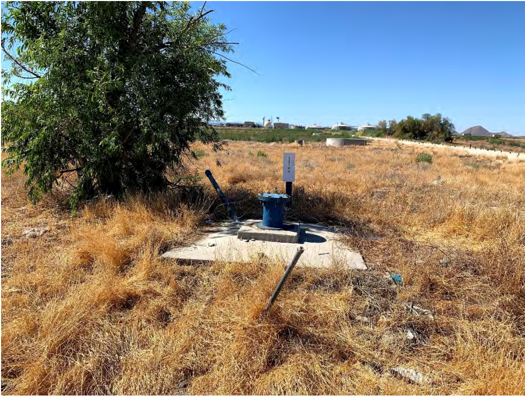
G-27. Groundwater irrigation well at eastern boundary of Site (08/03/2021)
