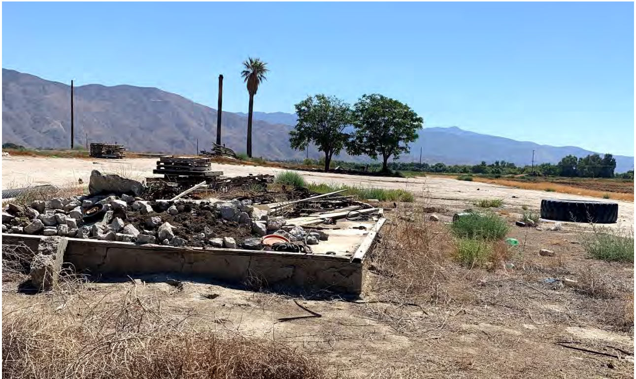
G-26. 15-foot by 10-foot concrete foundation and debris southwest of residence area (08/03/2021).
